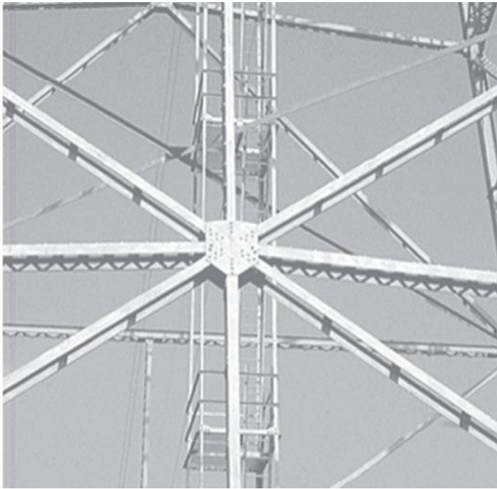
Gusset plate used to connect eight members
