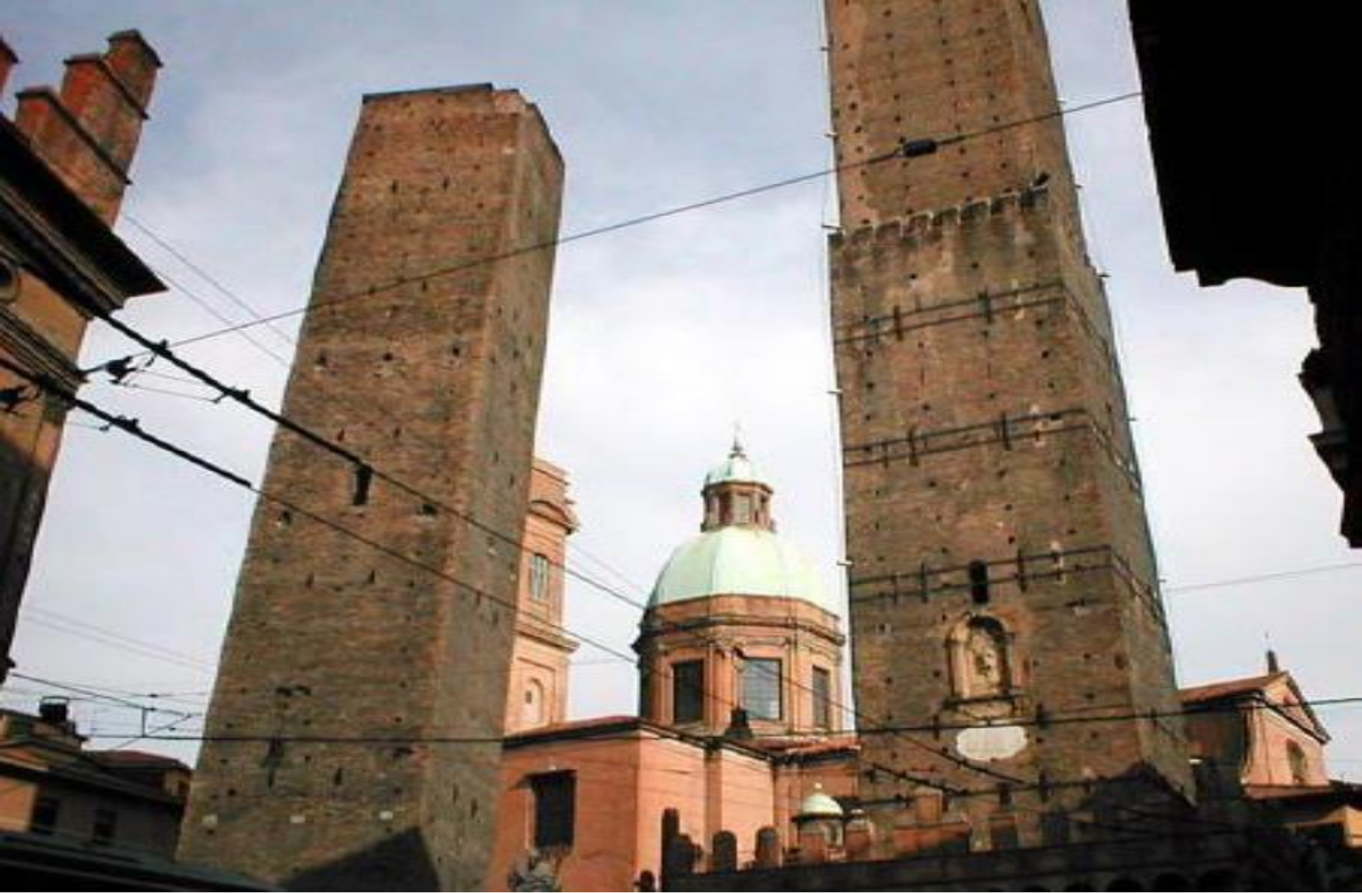
Tilting of Garisenda Tower (left) in Bologna, Italy (built in 12 th 5 Century)
