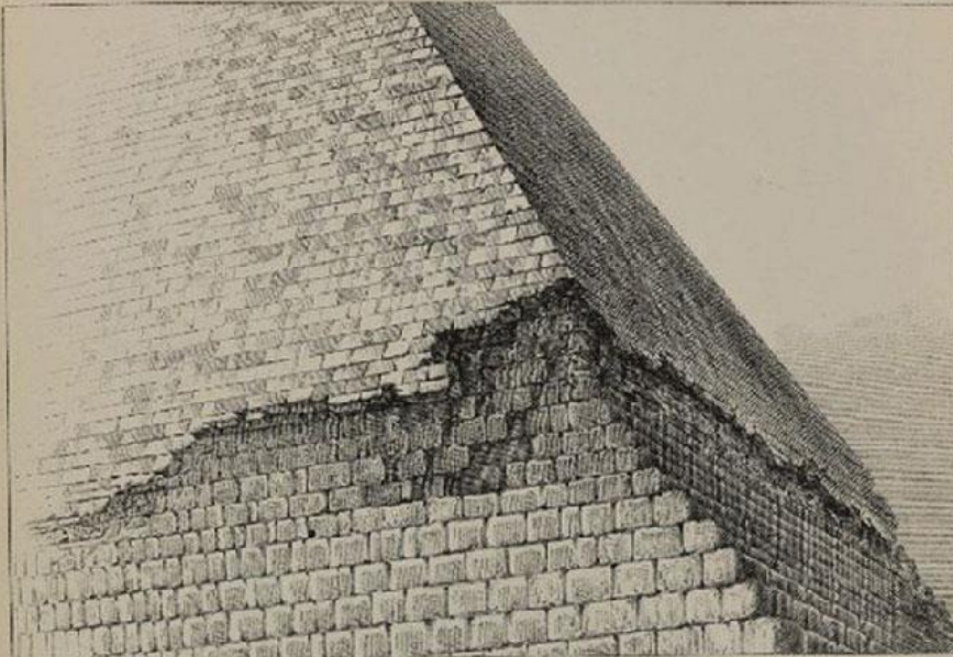
EXAMPLE OF THE CASING-STONES OF A PYRAMID. SUPER-POSED. ON THE RECT-ANGULAR MASONRY COURSES: FROM A PHOTOGRAPH BY P.S. OF THE SUMMIT OF THE 2 d PYR.
