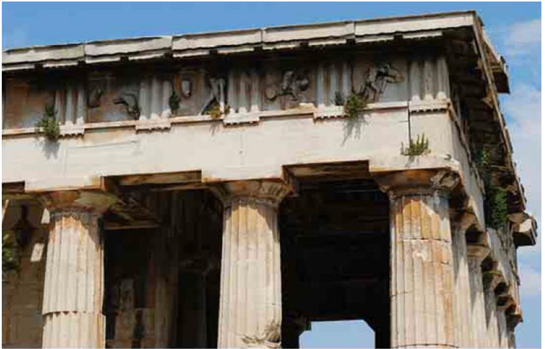
The entablature showing the architrave, frieze with triglyphs and metopes and the overhanging cornice
