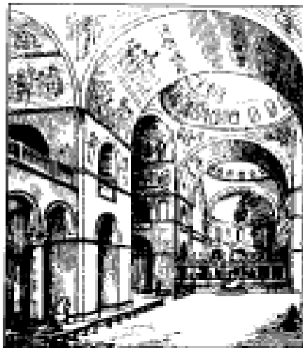
F INTERIOR OF S-MARK LOOKING E.
