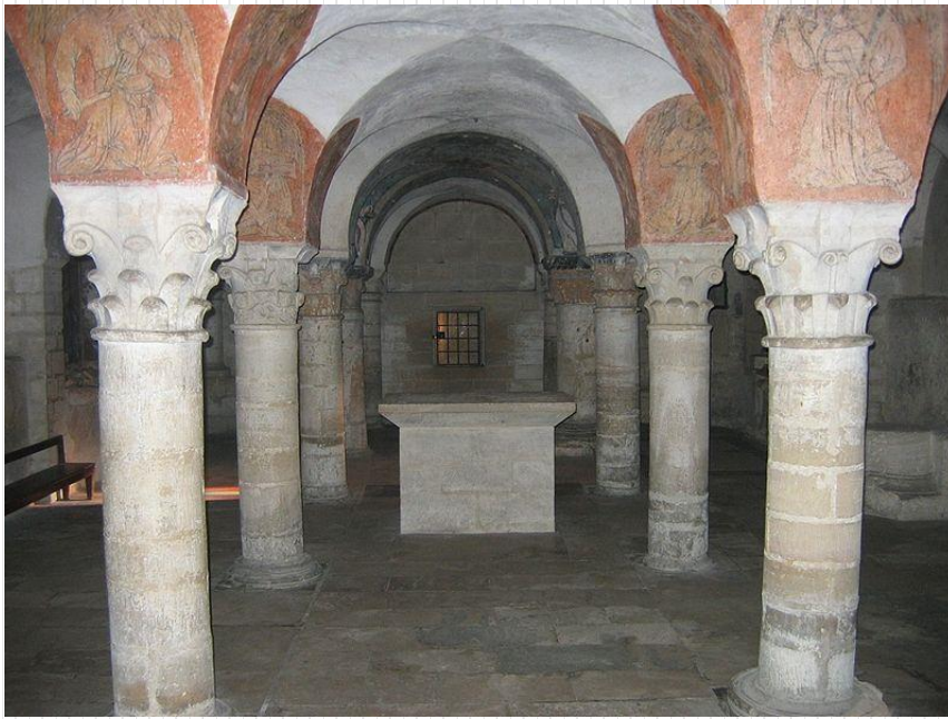
Bayeux Cathedral, the crypt has groin vaults and simplified Corinthian capitals.
