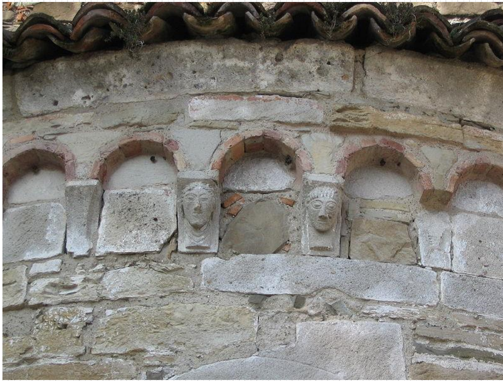
A Lombard band is a decorative blind arcade, usually exterior. A Lombard band in the Basilica di Santa Giulia, northern Italy.
