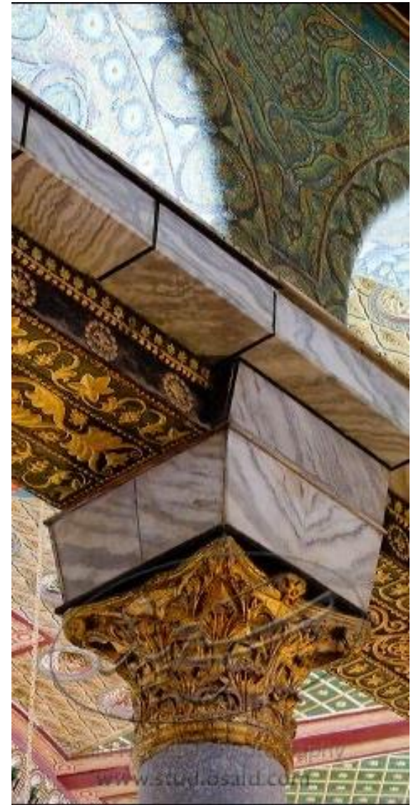
Column detail, Dome of the Rock
