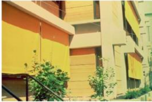
Figure 9.4k The automated fabric roller shades on the exterior of east and west windows are guided by vertical support cables which keeps the shades from swaying in the wind.
