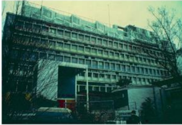
Figure 9.1j Sunshades known as brise-soleil were retrofitted on the Cité de Refuge, Paris, which Le Corbusier designed in 1932 without sunshades. (Photograph by Alan Cook.)
