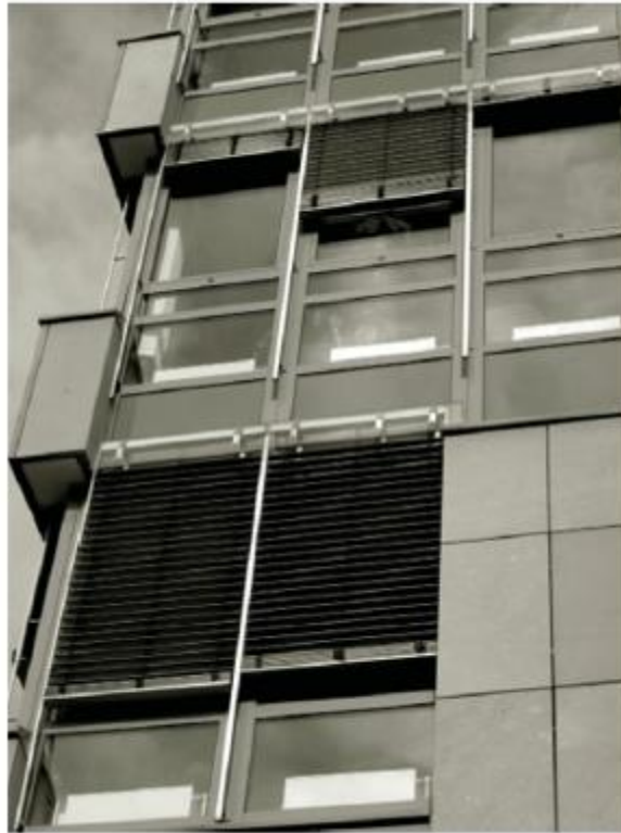
Figure 9.4n Exterior venetian blinds have all of the adjustments possible with interior venetian blinds, but they are much more effective in keeping the sun out. They also make an architectural statement on the facade. This building is in Freiburg, Germany.
