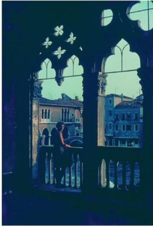
Figure 9.1d Loggias supported on arcades and colonnades shielded the large windows necessary for natural ventilation in the hot and humid climate of Venice, Italy. Sometimes an open-walled extra floor was added above the top floor to ventilate the heat collecting under the roof.
