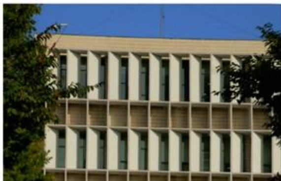
Figure 9.11d This photo of west facing windows was taken on a summer afternoon. The lack of shading by the vertical fins is proof of their impotence. Fins are not effective shading devices on east and west windows!
