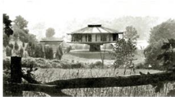
Figure 9.15b The residence that architect Richard Foster built for himself in Wilton, Connecticut, in 1967 is round and rotates 360° to take full advantage of the panoramic view and passive solar heating. (Courtesy of Richard Foster, architect.)
