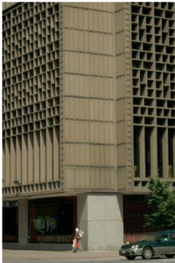
Figure 9.14c Small and medium-sized eggcrate shading systems severely block the view. Medium to large eggcrate systems are usually made of concrete, while small eggcrates are often made of masonry units.
