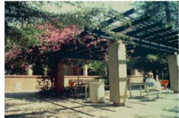
Figure 9.16g This pergola was designed so that most of the shade comes from the vine that it supports.
