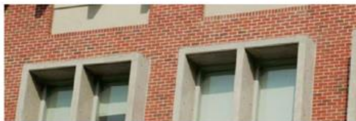
Figure 9.11f Since the depth of an overhang is a function of the height of a window, short window will require less deep overhangs.
