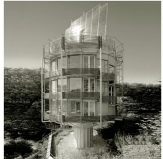
Figure 9.15c Architect Rolf Disch of Freiburg, Germany, has designed his home to track the sun. His Heliotrope house rotates to face welcoming windows toward the winter sun and a blank wall to intercept the summer sun. The PV panels on the roof rotate separately to always collect the maximum solar radiation. (Courtesy of architect Rolf Disch.)
