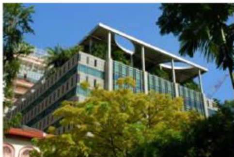
Figure 9.15i This parasol roof in Singapore shades both the actual roof and the roof garden.
