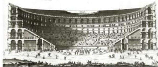
Figure 9.16b The Roman Colosseum, which was built about A.D. 80 and seated about 50,000 spectators, was covered with a giant awning for sun protection. (From Lanfiteatro Flavio Descritto e Deliniato , by Carlo Fontana, Vaillant, 1725.)
