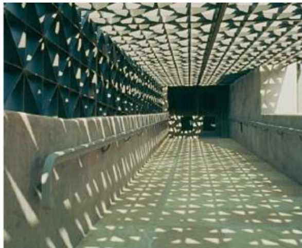
Figure 9.16i The typical pergola has shading elements that are on edge like joists. Such a design will provide little shade at 12 noon. Instead, the louvers should be tilted toward the north.
