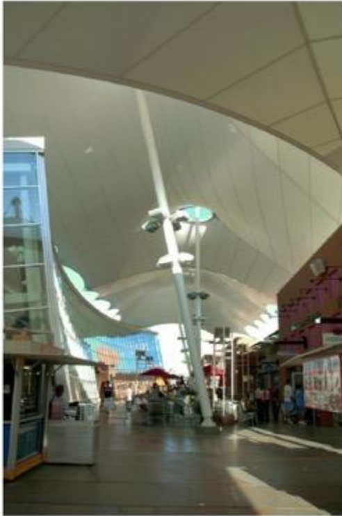
Figure 9.16a The public areas in this outdoor mall in Las Vegas are shaded by translucent membrane tension structures.
