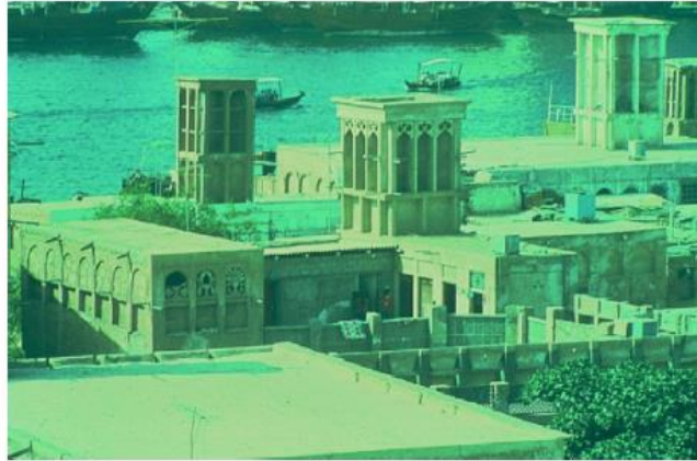
Figure 10.2d The wind towers in Dubai, United Arab Emirates, are designed to catch the wind from any direction. These substantial wind towers evolved from the one shown in Fig. 1.2d. (Photograph by Mostafa Howeedy.)
