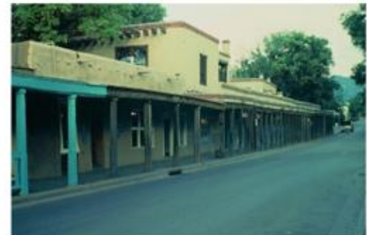
Figure 11.1e This colonnade in Santa Fe, New Mexico, protects pedestrians from rain as well as sun, and it shades the windows and walls.
